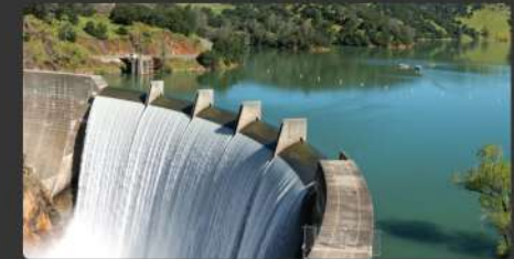
Lesotho Water Supply
