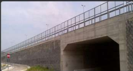
Albania Transportation Roads Bridges
